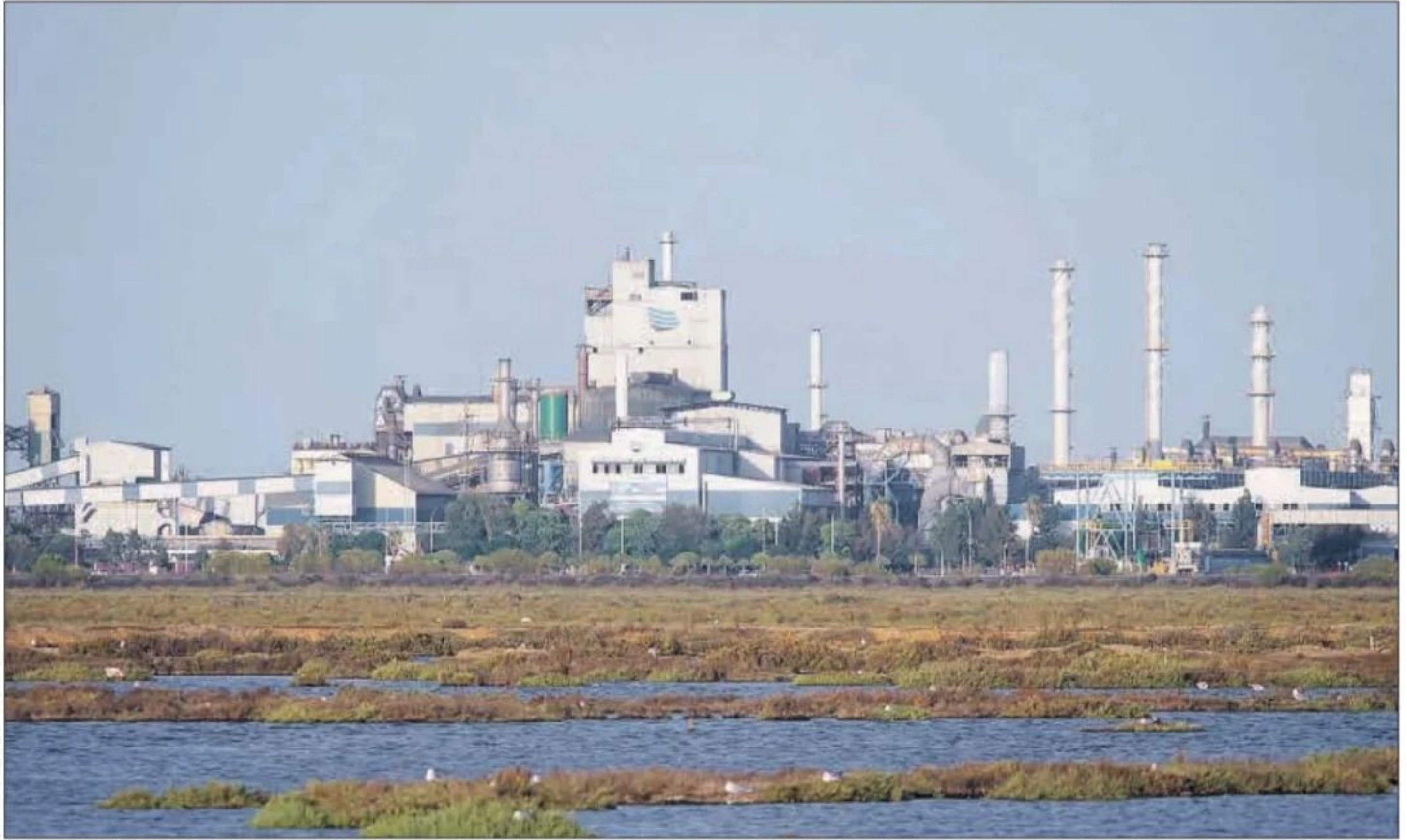
Fachada de Atlantic Copper. ATLANTIC COPPER.
